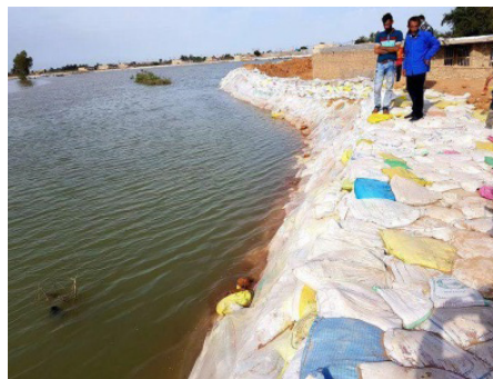
Picture 6 Damaging the riverbanks as a result of building levees Source: (Rahyab Press)
