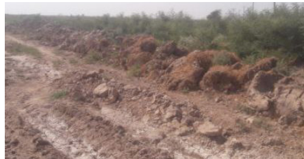
Picture 4 A levee left behind in the natural environment after the abatement of the flood Source: (Asr-e-Iran Daily)
