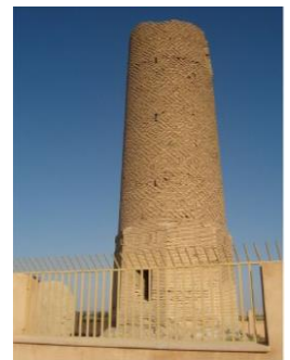
Figure 4. Gar Minaret Source: Autores
