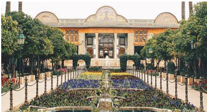
Figure 1. View of the northern building of the Qavam House building. Source: Authors.
