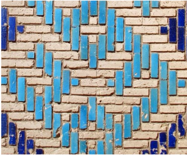
Figure 5. Display of details in the Ma'qelis of the Khargerd Ghiasieh School. As can be seen, the size of 5 squares is used with one brick (3 pieces) and one brick (2 pieces) without a joint between the bricks. Decoration under the porch of the side entrance from the west front to the mosque. Source: Author.
