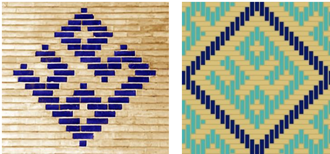
Figure 1. On the right, the word Muhammad with a simple brick arrangement, which only the color contrast of the bricks makes the design work. On the left, the word Muhammad with Khofte-Raste brick arrangement (redesigned decoration from the Khargerd Ghiasieh school). Source: Author.
