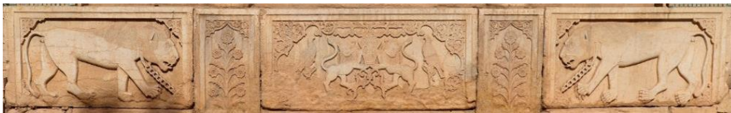
Figure 47. The plinth on the west side of Mohtasham house. Source: Authors.
