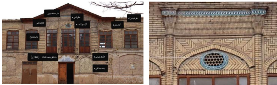
Figures 19 & 20. Brickwork and tiling decorations on the exterior of the eastern side of Mohtasham house.
