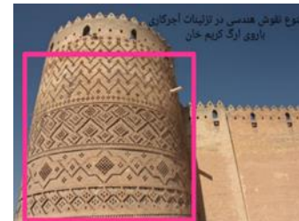
Figure 8. Types of geometric motifs in the brickwork decorations of Karim Khan Citadel rampart, Shiraz, Zandiyeh. Source: https://commons.wikimedia.org/
