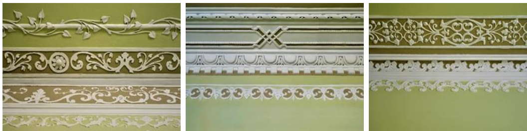
Fig 12. Stucco motifs on the ceiling of the bedrooms on the second floor. Source: Authors.
