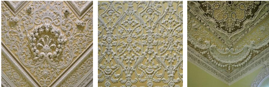
Fig 10. Applying high-relief and semi-relief techniques on the ceiling of different interior spaces of the building. Source: Authors.
