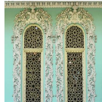
Fig 9. Stucco motifs on the margins of the doors and windows of the exterior of the house. Source: authors.
