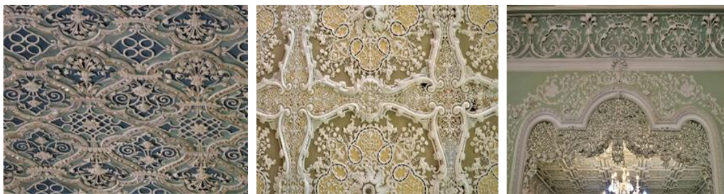
Fig 11. Stucco on the flat mirror on the wall and ceiling and combining the art of mirror work and stucco on the porch ceiling. Source: Authors.
