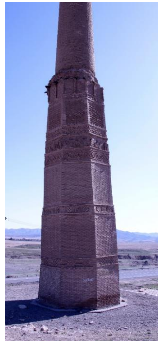
Fig 3. Karat Minaret, the west side of the minaret Source: Authors.
