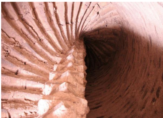
Fig 6. The core of the second part of Karat Minaret. Source: Authors.
