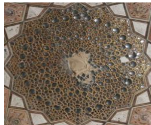
Fig 2. Cupbori, ceiling of Hasht Behesht building. Source: Authors.
